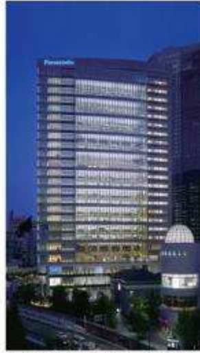
Panasonic Tokyo Shiodome Building (Tokyo, Japan)
