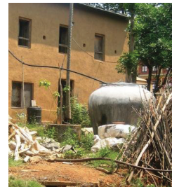
Rain (roof) water harvesting
