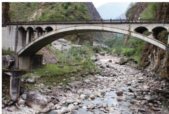
A remnant of the small stone bridge (on the left) destroyed by the glacial lake outburst flood of 1981 –the Zhangzangbo glacial lake lies about 27 km upriver in the Tibetan Autonomous Region of China
