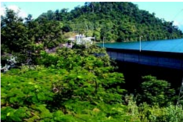
Photo 3.5 Num Ngum Dam, Vientiane Province
