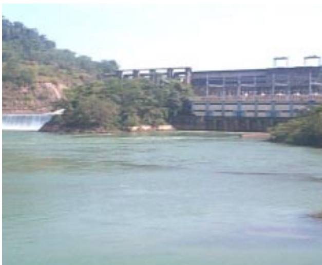
Photo 2.1 Num Ngum Dam, Vientiane Province
