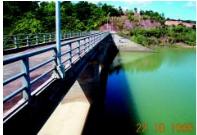
Photo 3.4 Xong River Diversion Canal to Num Ngum Reservoir, Vientiane Province
