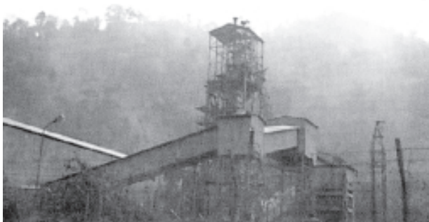
Photo 10.2 Fugitive emissions at a limekiln unit
