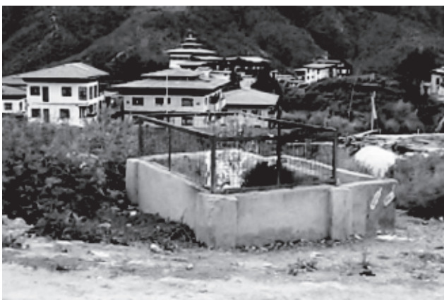
Photo 12.3 Garbage container in Thimphu
