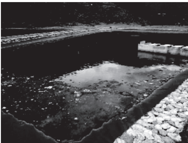
Photo 11.5 Sewage treatment plant
