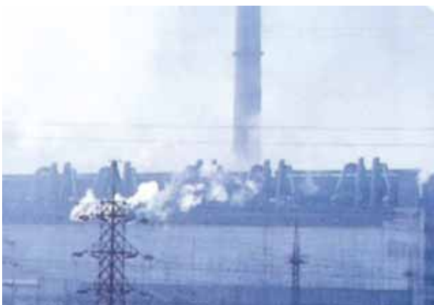
Photo 3.11 Pyongyang thermal power plant
