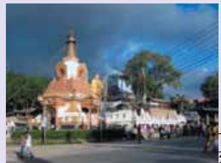
New statues and stupa being constructed on the western side of Swayambhu hill
