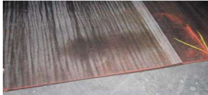
Figure 8 Enhancement of a concrete floor by application of impermeable flooring (source: DNSC)
