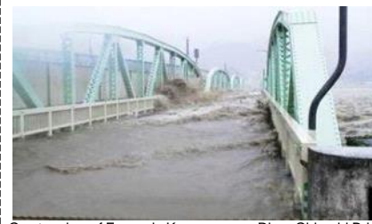
Overtopping of Formerly Kumanogawa River Ohhashi Bridge (photo taken from the right bank)
