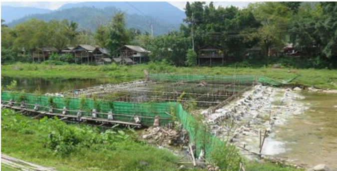
An example of ecosystem-based adaptation measures: Living weir
