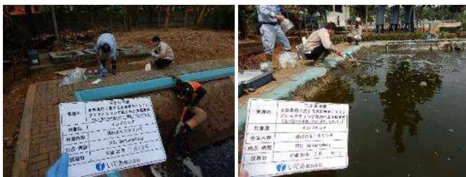
Figure 4.1-3 Pictures of water monitoring demonstration
